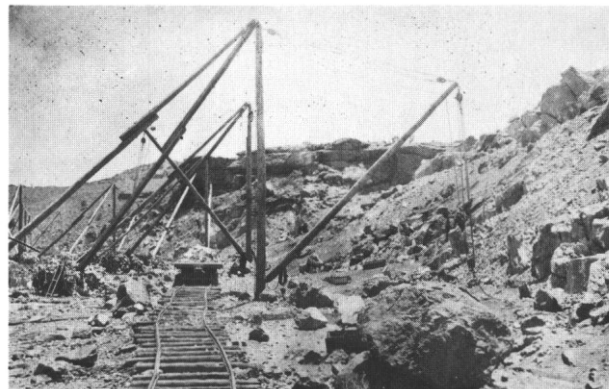
Quarrying limestone along San Pedro (Carthage) branch, AT&SF Railway, ca. 1884. Both steam "donkey" engine and mules were used to snake limestone boulders onto flatcars which were then hauled to Socorro for flux at the smelter. Joseph E. Smith photo, courtesy Ed. Smith.
